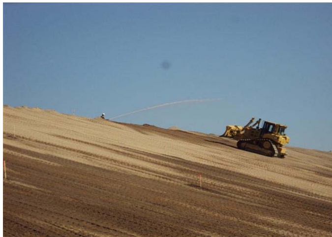
CAMU: Track walking the first lift of cover soil on the south slope of Phase 2.
