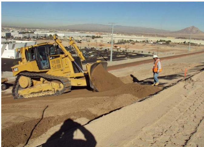
CAMU: Phase II, West slope, final cover soils.
