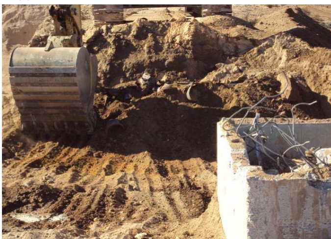
Eastside, Southern rib berm removal.
