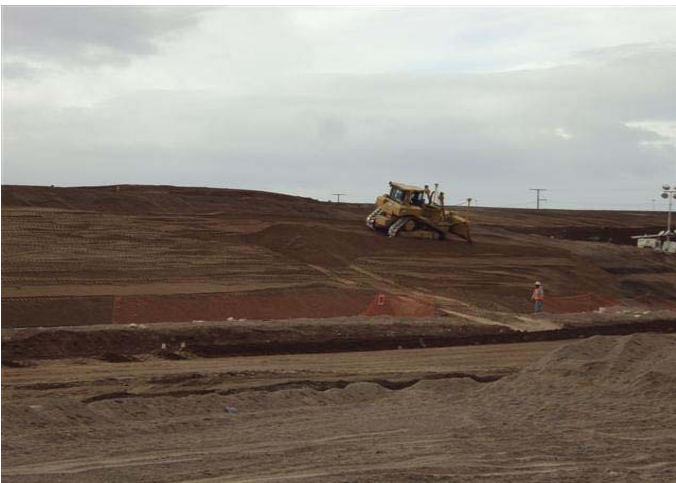
CAMU: Phase IV, north slope, interim cover placement.
