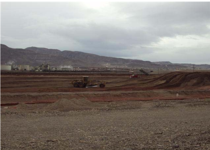
CAMU: Phase V, waste placement.
