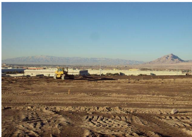
CAMU: Phase II, interim cover installation.
