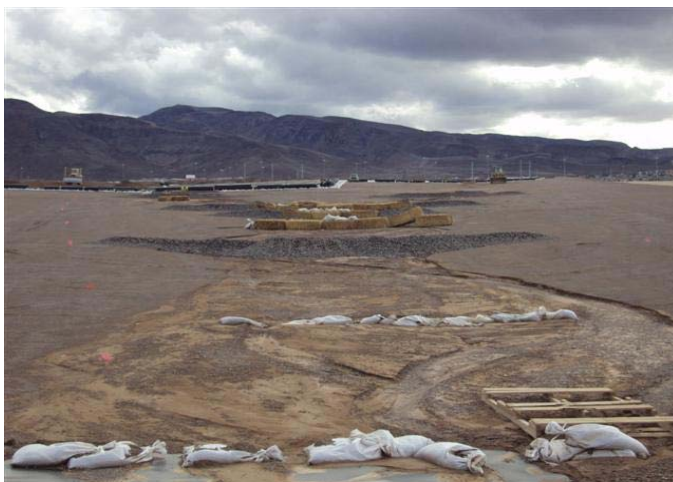
CAMU: Phase I and Phase II, temporary check dams.
