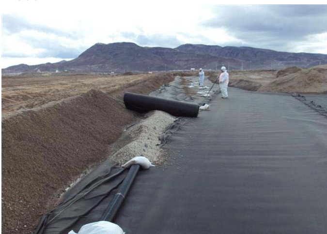
CAMU: Phase I and Phase II, top, LCRS Pipe installation.
