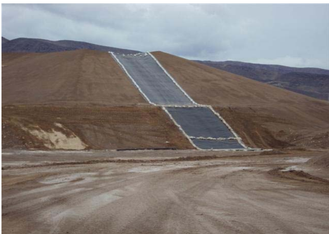
CAMU: Phase IIIB, North slope, placed for temporary storm run off.
