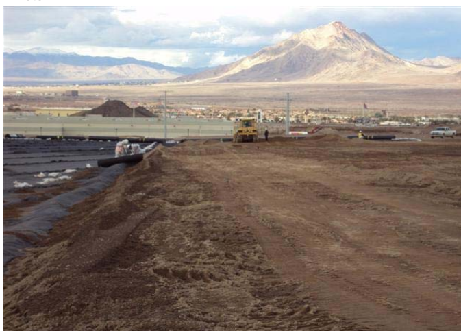
CAMU: Phase II and Phase I, LCRS pipe installation and final cover soils.
