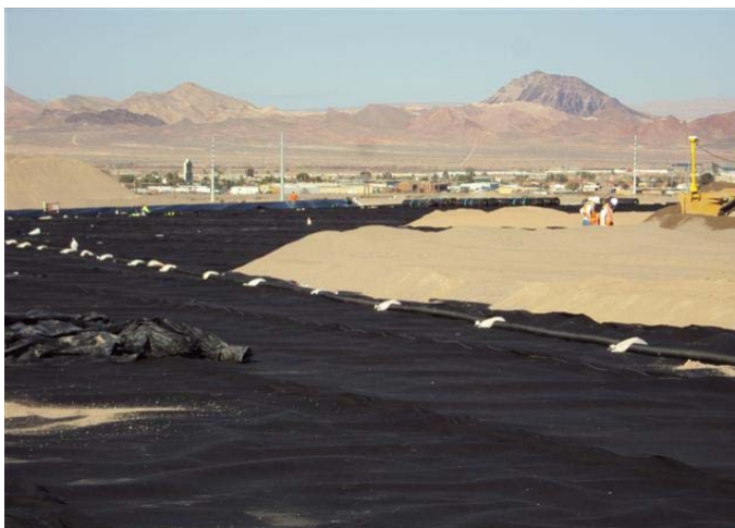
CAMU: Phase I and Phase II, placing final cover soils.
