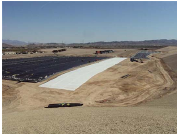
CAMU: BMI North, geosynthetic installation.
