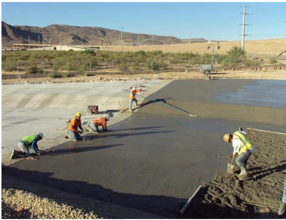
CAMU: South west channel, concrete pouring and finishing.
