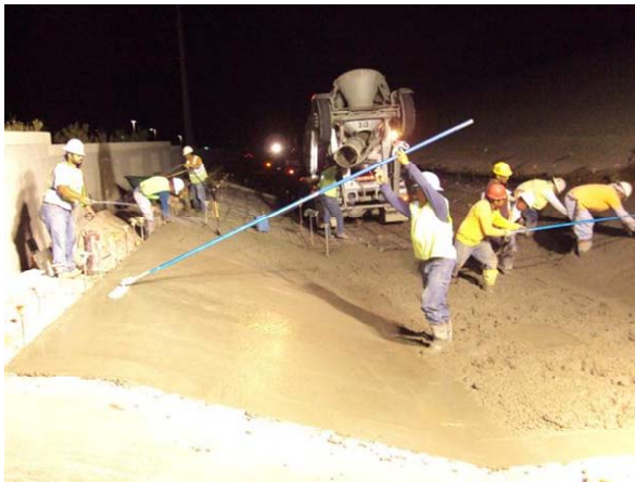
CAMU: West channel, concrete pour and finishing.
