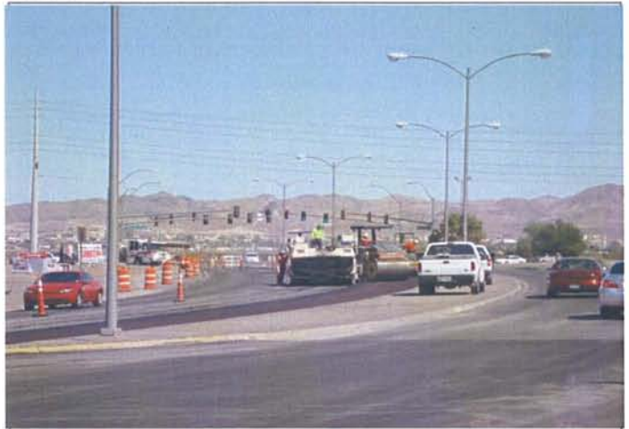
Westside: Westbound West Warm Springs Rd. Paving overlay..
