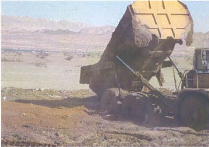
Eastside: Dumping wet soils in dry ponds.
