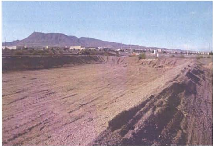
Eastside: Debris Lined Storage area subgrade being worked.
