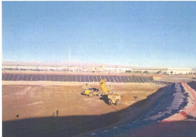
CAMU: Phase 1 western ditch soils dumping.
