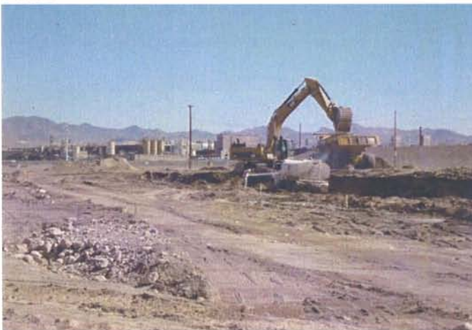
CAMU: Phase 111A, Western ditch being excavated.
