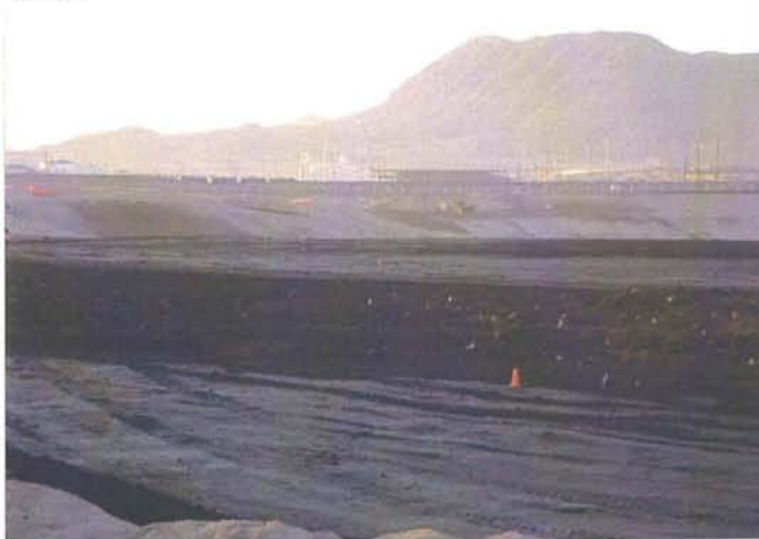
CAMU: Rejected lift in phase I being reworked.
