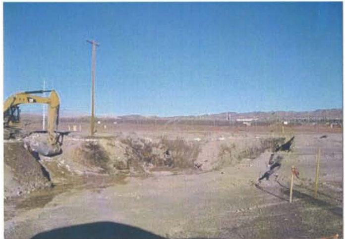
CAMU: Northeast Equalization Basin, chasing impacted soils and debris.
