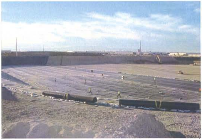
CAMU: Phase II liner installation looking west. Western ditch, west slope being rolled.
