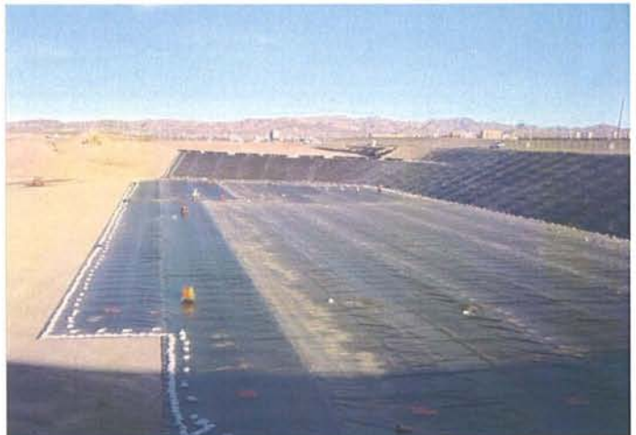
CAMU: Phase II liner being installed on floor.
