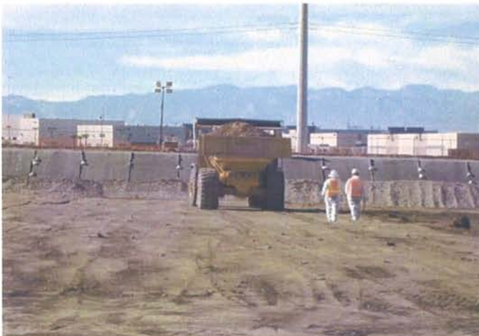
CAMU: Phase I proofrolling on waste monitored by Geosyntec personnel.
