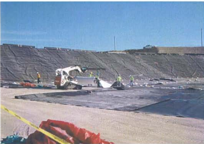
CAMU: Phase II, GCL Liner being installed.
