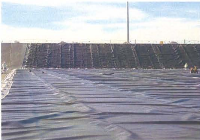
CAMU: Western ditch liner, West slope and floor.
