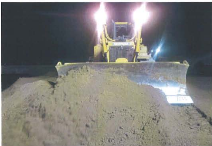
CAMU: D6 Dozer pushing and placing operations layer.
