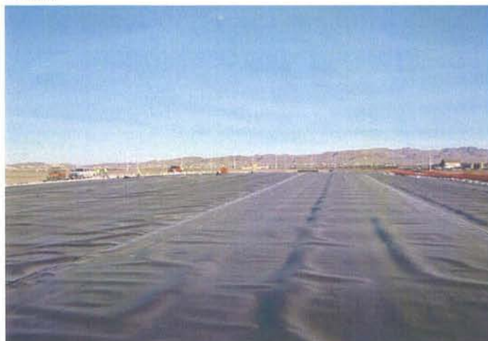
CAMU: BMI North Landfill Liner deployment, looking east.
