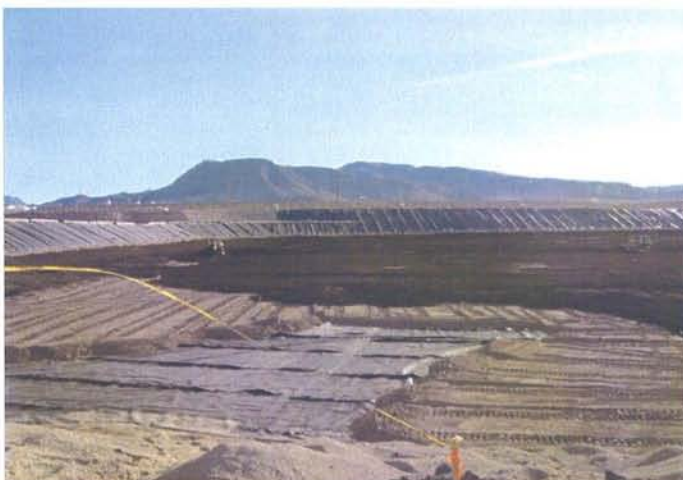
CAMU: Phase II last area covered by operations layer.
