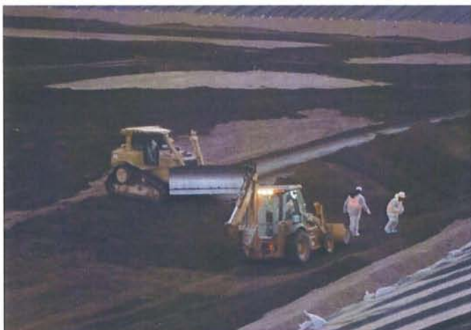
CAMU: Phase II, operations layer placement, watching for oversized material.
