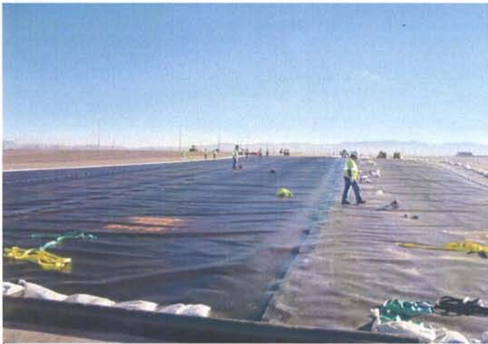
CAMU: BMI North Landfill Cap liner installation continues.
