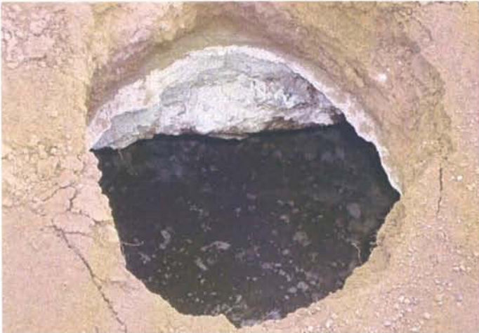
CAMU: BMI North Landfill Cap, Sink hole found while compact rolling.
