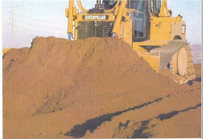
CAMU: BMI Landfill North, first lift pushout.
