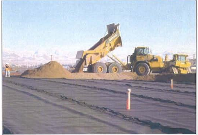
CAMU: BMI North Landfill, placement of 1 inch minus.
