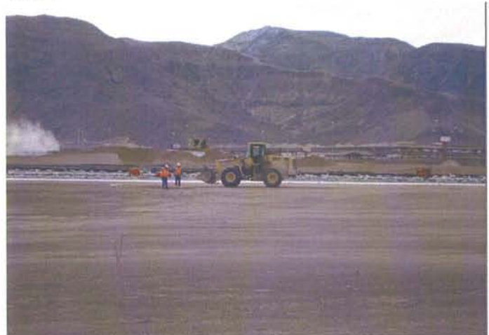
CAMU: North BMI Landfill subgrade preparation.
