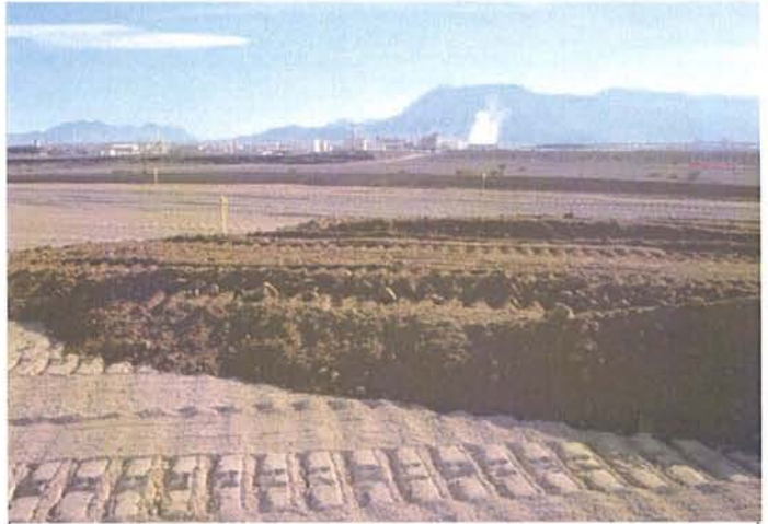
CAMU: North BMI Landfill second lift 6" minus placement.
