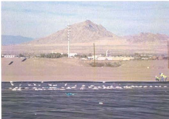
CAMU: North BMI Landfill geosynthetics, installation.
