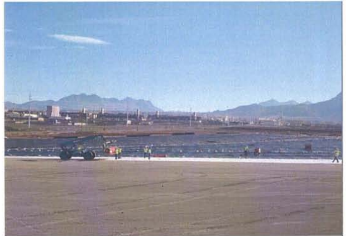
CAMU: North BMI Landfill geosynthetics, installation.
