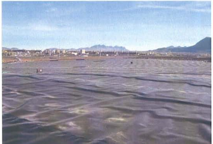
CAMU: North BMI Landfill liner installation, looking south.
