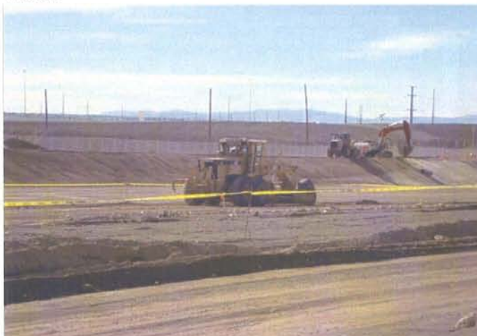
CAMU: Phase IIIA, subgrade preparation for liner.
