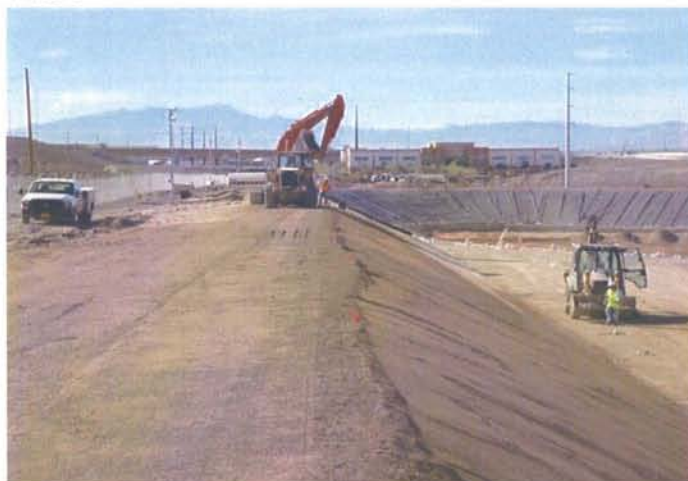
CAMU: Phase IIIA south slope preparation for liner.
