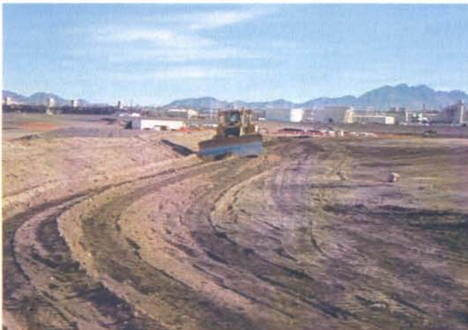
CAMU: Phase I top of waste, cutting in temporary berm.
