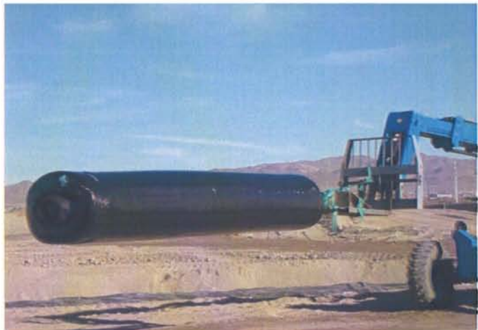
CAMU: Unloading geocomposite rolls with all terrain forklift and stinger bar.
