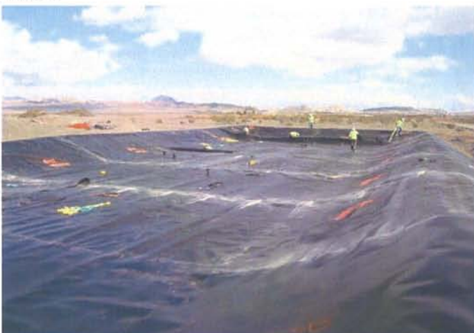
Eastside: Debris Storage area. Liner installation.
