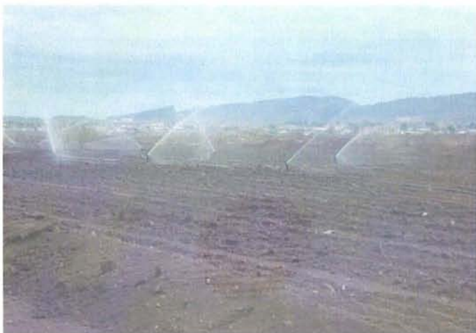
Eastside: Beta ditch, moisture conditioning with sprinklers.
