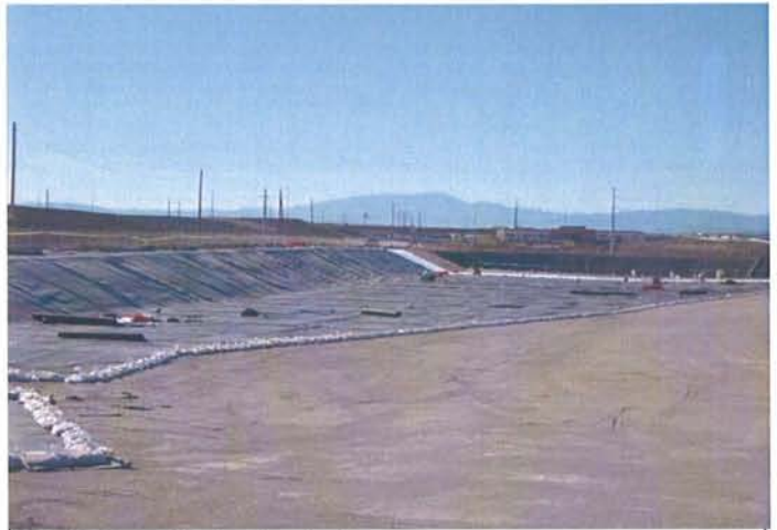
CAMU: Phase IIA Liner installation.
