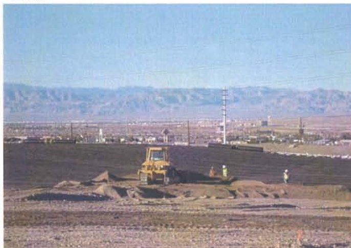
CAMU: Placing 1" soils on North BMI Landfill.
