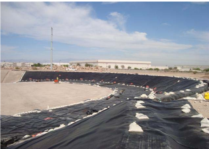
CAMU: Phase IIIB. Liner installation.
