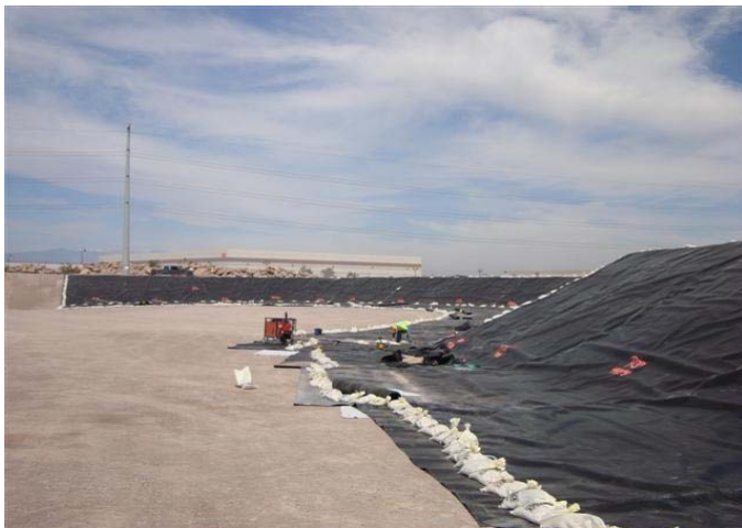
CAMU: Phase IIIB, Liner installation.
