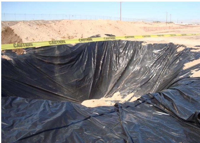
CAMU: SE-2, lined for PCB staging.
