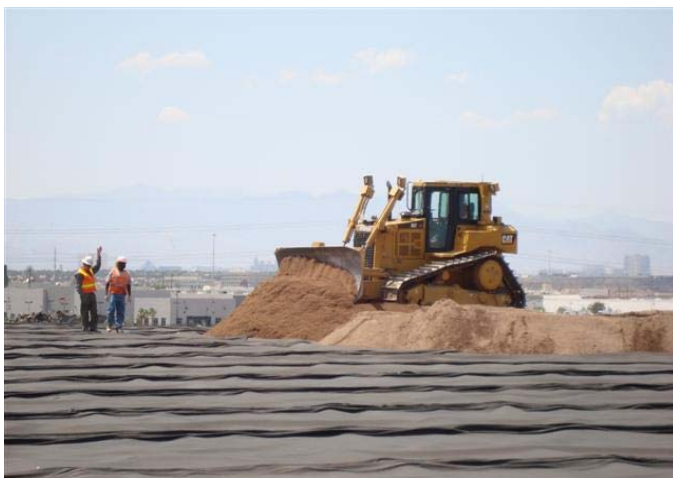
CAMU: Pushout of the 1-inch minus on BMI South Landfill.
