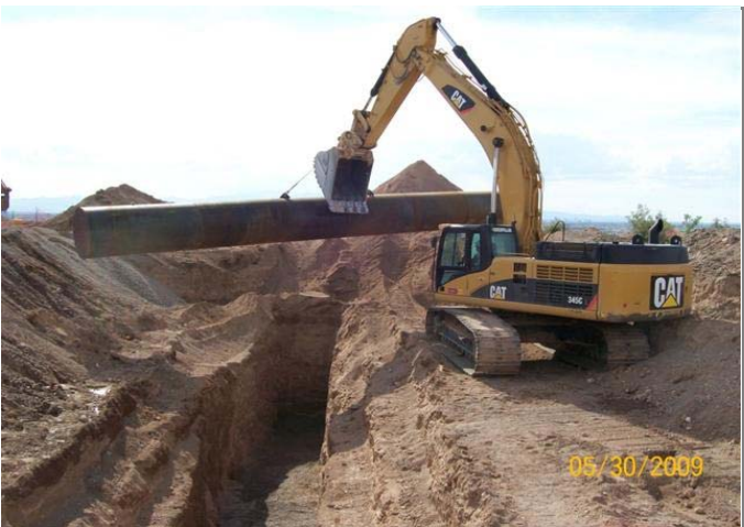
Eastside: Pipe casing.
