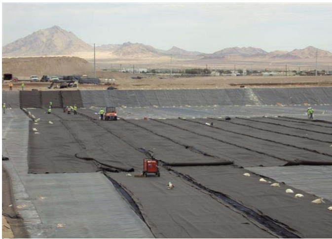
CAMU: Phase IV geocomposite deployment.
