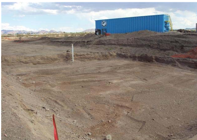
Eastside: 50' X 50' soil removal in sewer alignment corridor.
