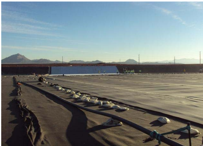
CAMU: Phase IV, liner installation.
