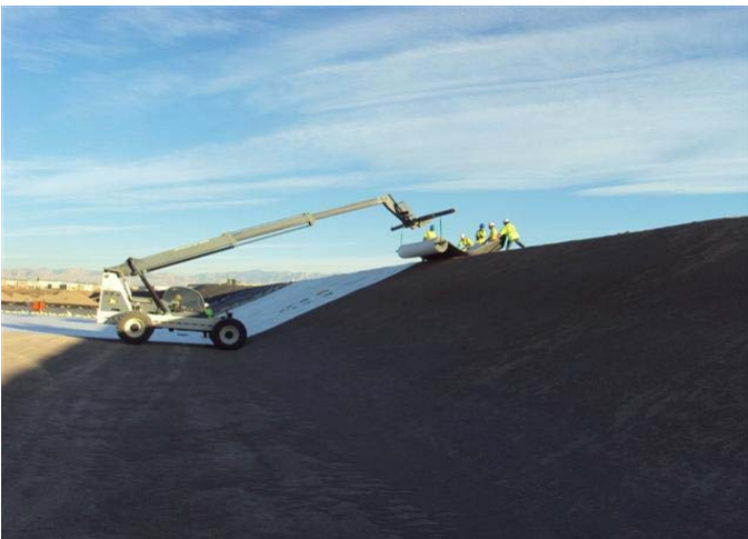
CAMU: Phase IV, liner deployment.
