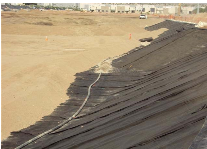
CAMU: Phase IV, LCRS pipe installation.
