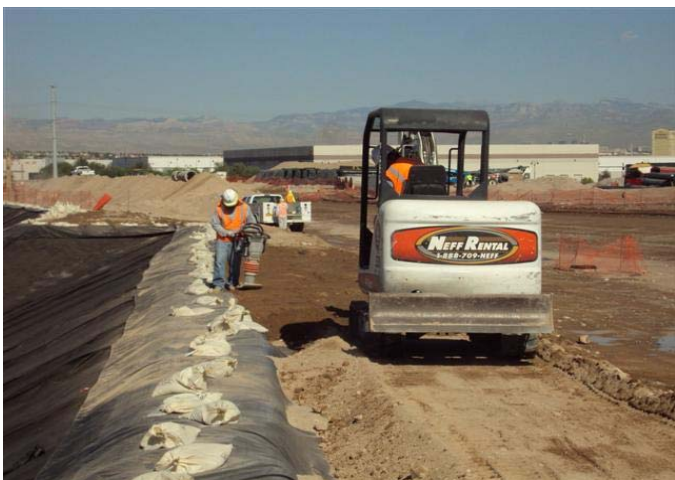
CAMU: Phase IV, Anchor trench backfill.
