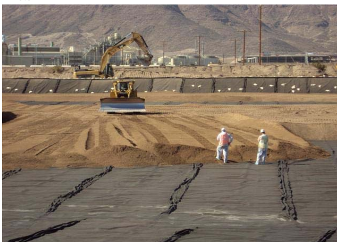
CAMU: Phase IV, operations layer placement.
