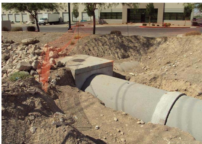
CAMU: 60" RCP storm drain pipe outlet to Manhole #8.
