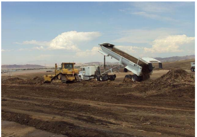
CAMU: Phase II, Shredded wood mixing and placement.
