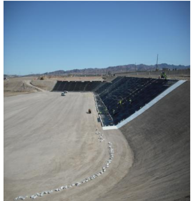
Liner Installation
