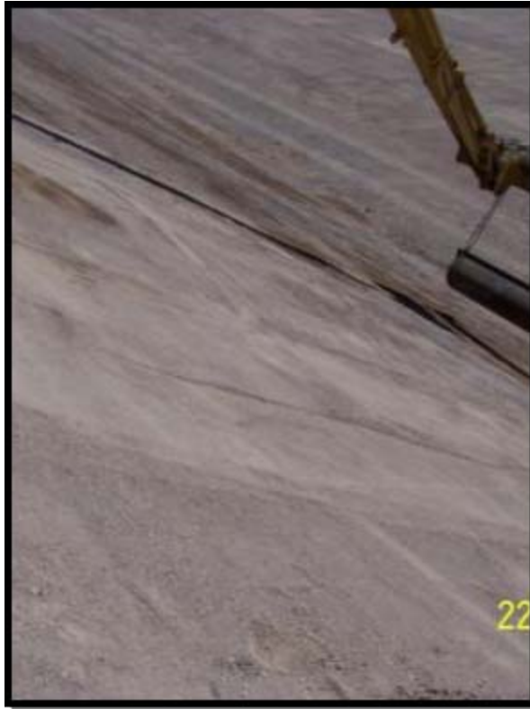
Subgrade Slope Compaction
