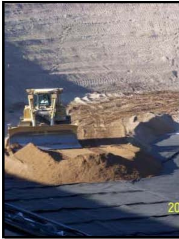
Placing & Spreading Operations Layer
