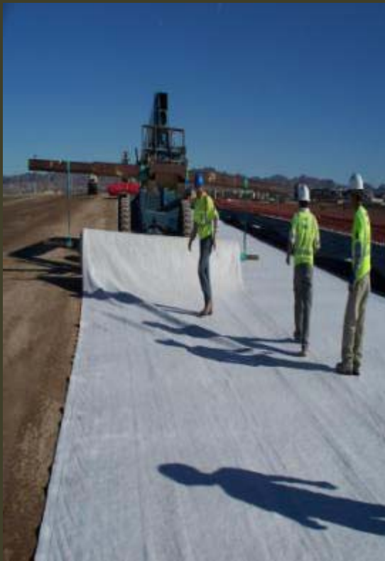
Geosynthetic Clay Liner Installation
