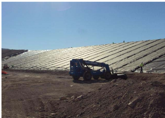
CAMU: Phase I and Phase II, east slope. Geocomposite liner placement.
