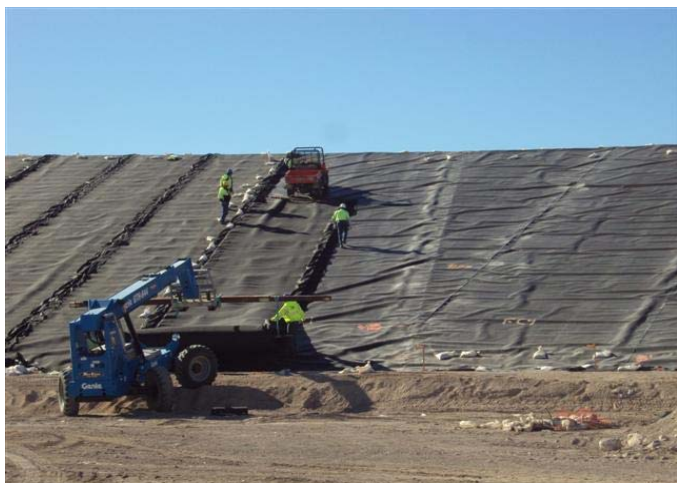
CAMU: Phase I and Phase II, east slope geocomposite layer.
