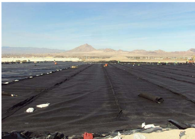
CAMU: Phase I and Phase II top, geocomposite.
