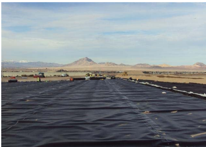
CAMU: Phase I and Phase II, geosynthetics.
