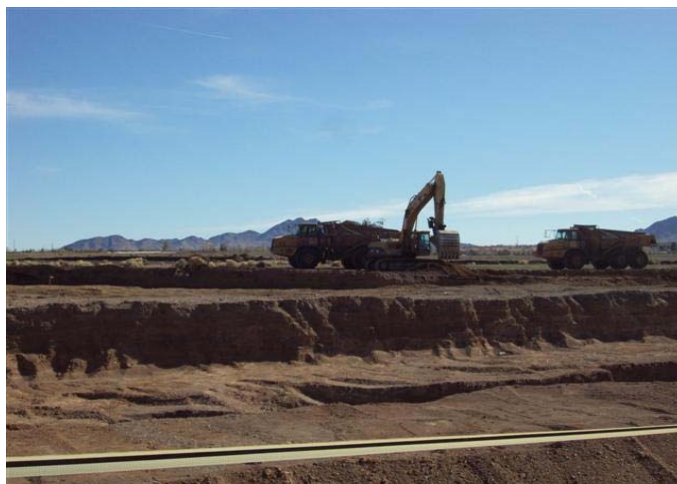
Eastside: Removing overburden in triangle at southern rib.
