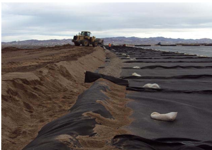
CAMU: Phase IV, CPE pipe and drainage rock.
