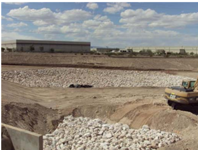
CAMU: Northwest Basin, riprap installation.
