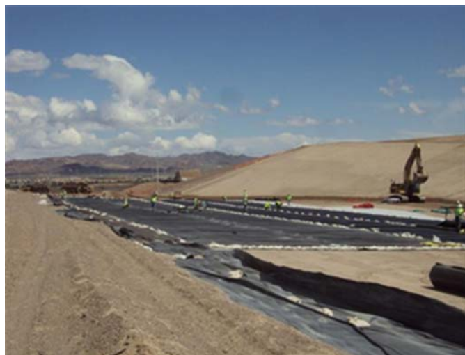
CAMU: BMI North, south perimeter, geosynthetics.
