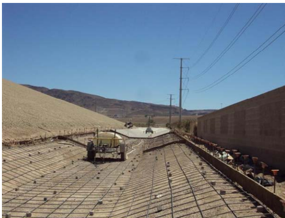
CAMU: West channel, concrete preparation.
