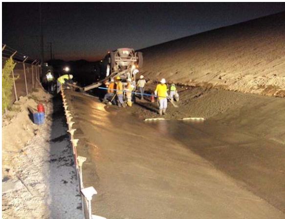
CAMU: West channel, concrete pour and finishing.
