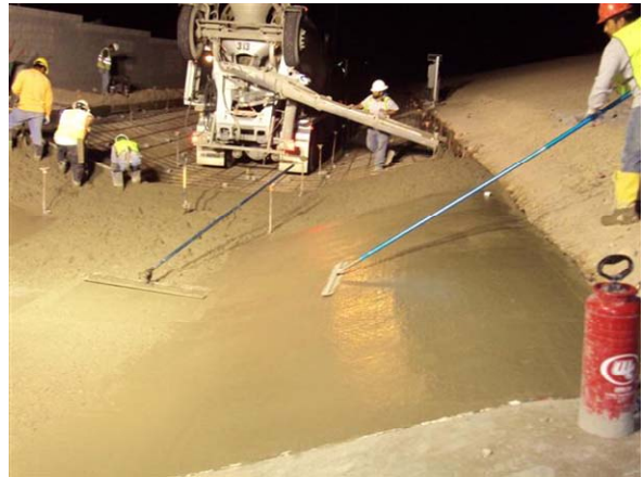
CAMU: West channel, concrete pouring and finishing.
