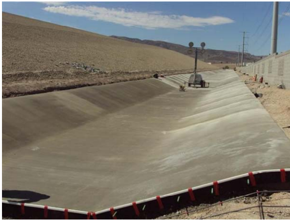
CAMU: West channel, concrete finishing.
