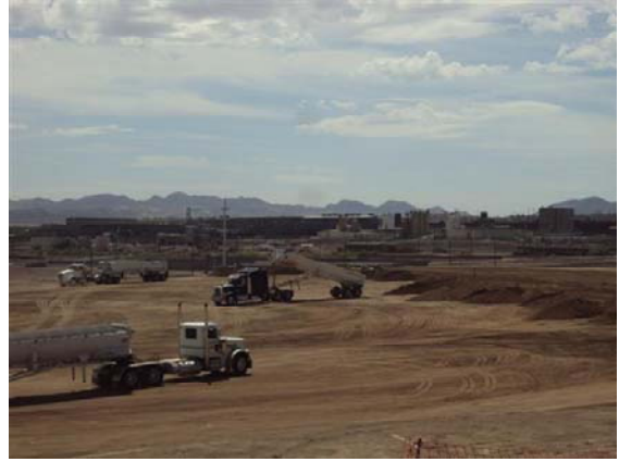
CAMU: Phase V, waste placement.
